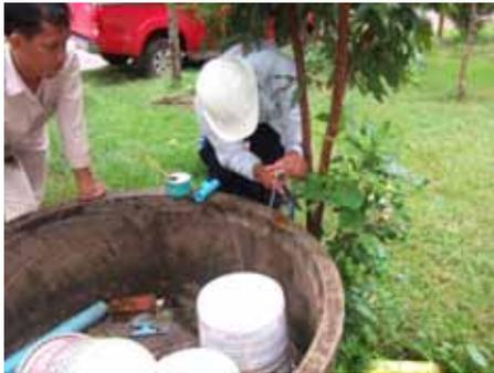
Pressure gauge installation for pressure 24 hours pressure test reading
